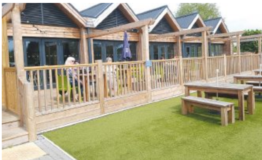
Large permeable paved area outside.
