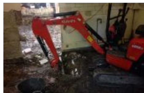
The rebuild involved excavating and 'tanking' the whole of the ground floor
