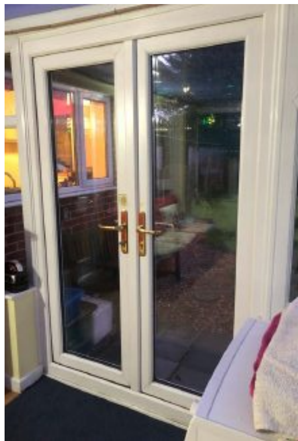
Flood resilient patio doors have been installed.
