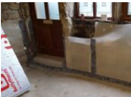
Waterproof membrane during installation.
