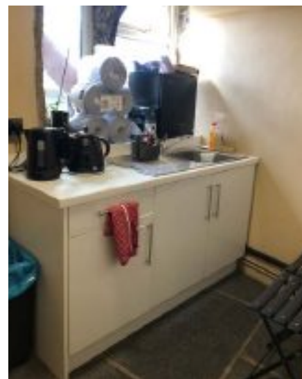
A plastic kitchen was installed.
