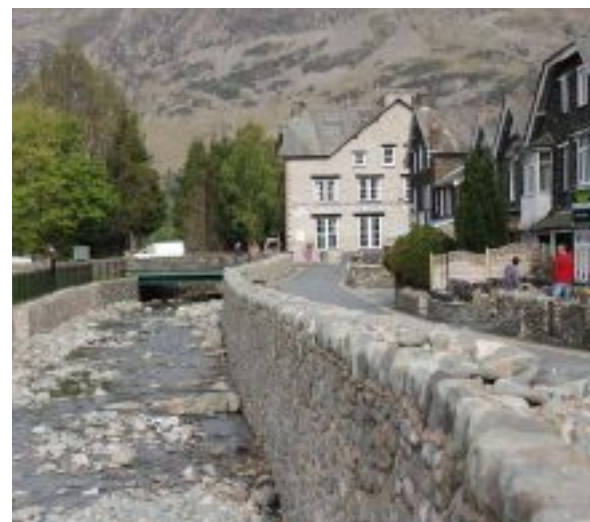
Newly upgraded Environment Agency defences.
