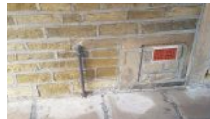
Walls were repointed and coated with a water proof spray and self-closing airbricks fitted.
