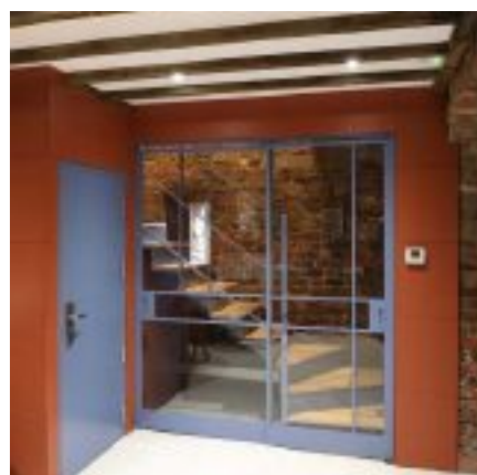
Glazed sliding door/screen in powder-coated steel.
