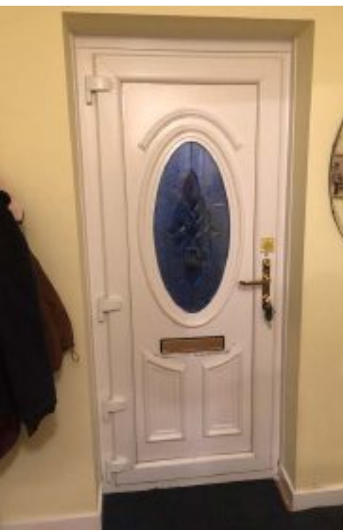
Flood resilient front door has been installed.
