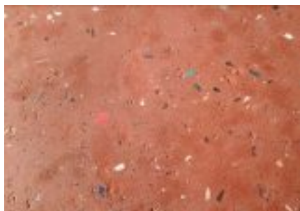
The walls were rendered using coloured renders.
