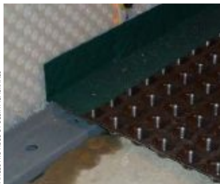
The 3mm floor membrane is also designed as an underlay for protecting oak floors.
