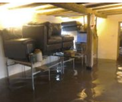
Furniture raised on tower scaffolding.
