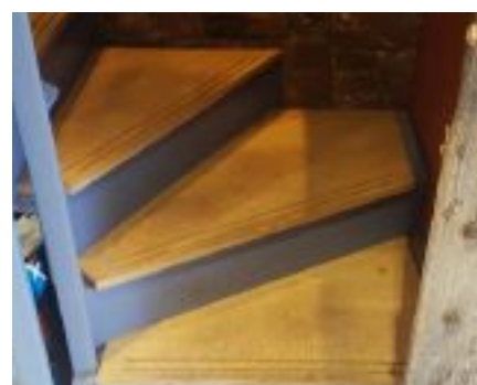
Steel staircase and solid oak treads.
