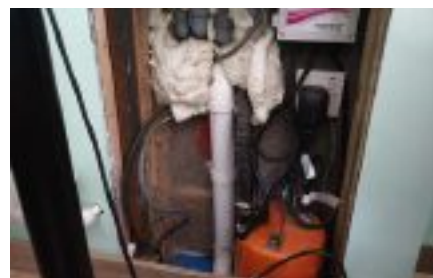
Sub-floor automatic high-performance skimmer pump.
