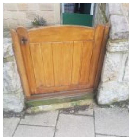
New wall at front of house with a flood-proof gate
