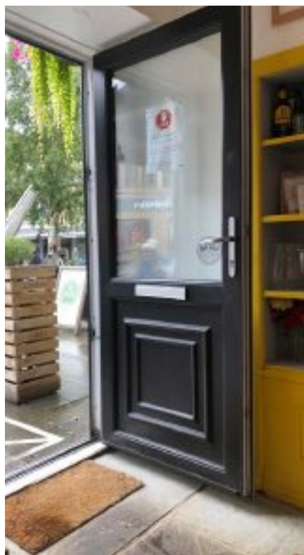
Kitemarked flood door and stone flagged floor.
