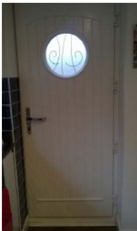
Flood resilient doors have been installed.
