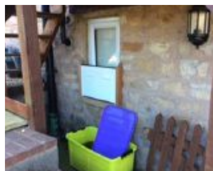
Flood barrier to basement door and window.
