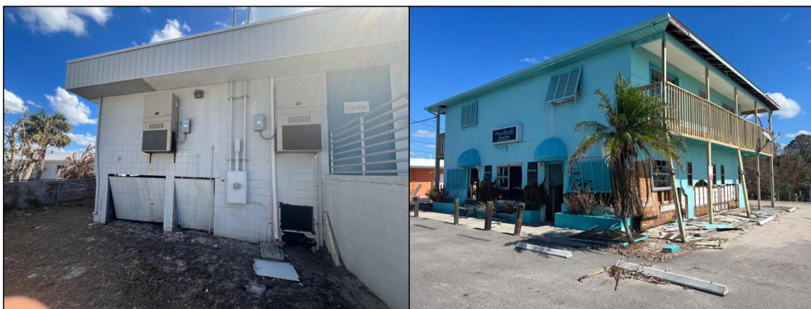
Figure 8: Low-rise commercial buildings, near the coastline, suffered damage to exterior walls and windows due to storm surge in Manasota Key.
