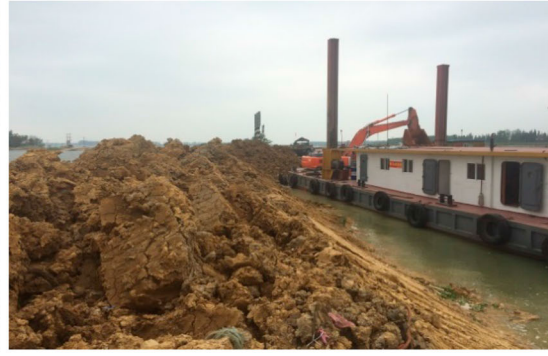
(b) Breach of Yaobu Polder was blocked with shipped soil
