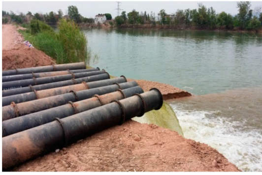
(a) Draining after the breach was blocked in Wuqi Polder, Zongyang county.
